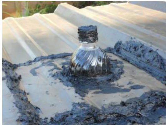
Fig.2 Installation of Solar Bottle Bulb
