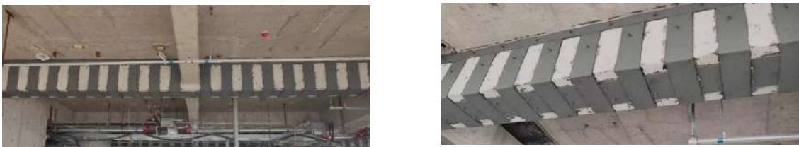
Figure 6 Plate bonding in structures
