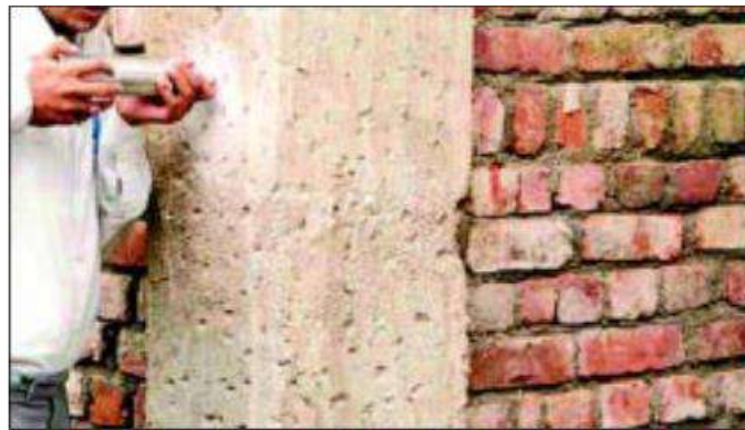
Figure 7 Rebound hammer test being performed on a column.
