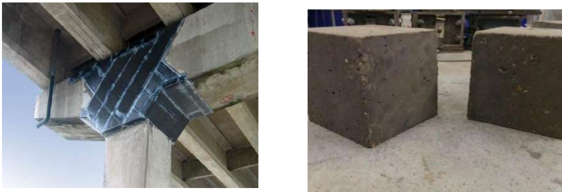
Figure 3 Polymer concrete cubes and its use in column fills.
