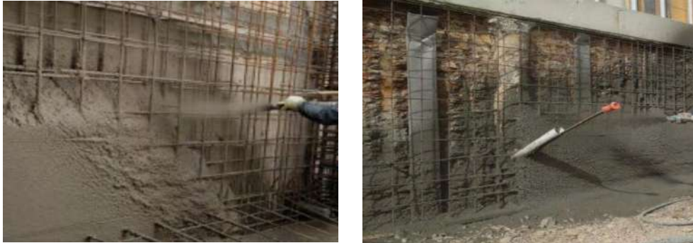
Figure 1 Application of shotcrete
