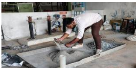
Figure 5.1: Mixing of Concrete
