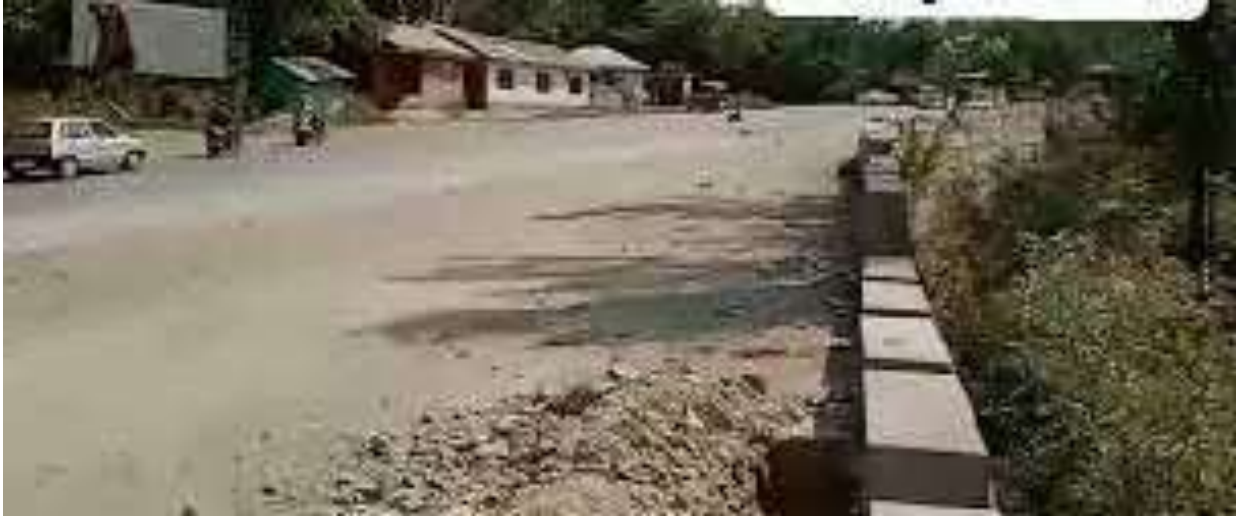
Figure 2 Road construction at Nagbal Ganderbal
