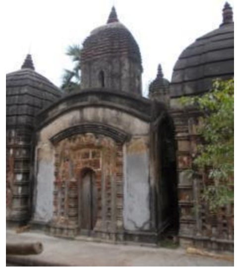
Pancharatna temple of Jalandi pic - 5
