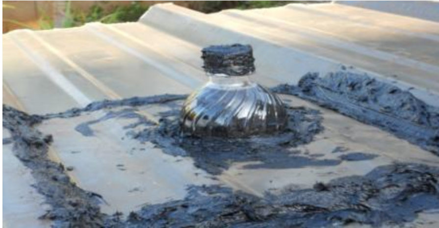
Fig.2 Installation of Solar Bottle Bulb
